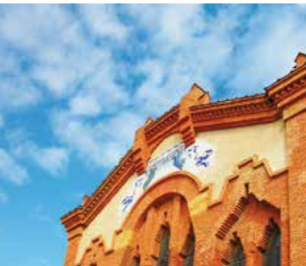
Pinell de Brai, Cooperative Wine Cellar
